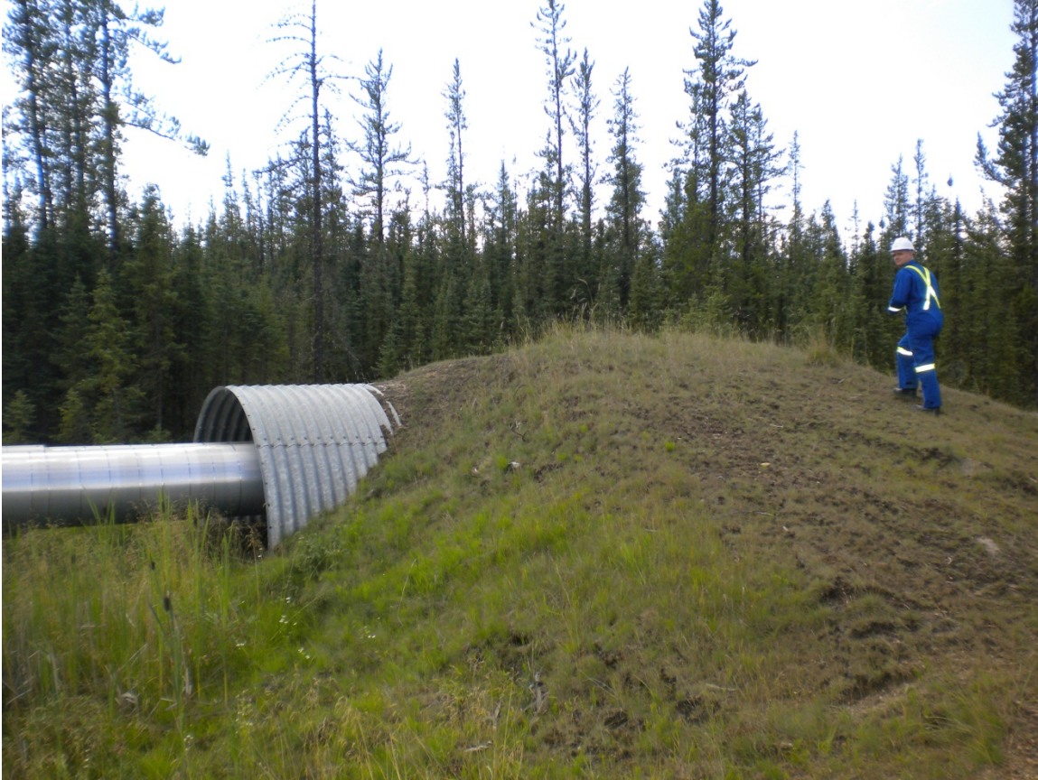
Figure 3. Culvert crossing structure in northeast Alberta.
